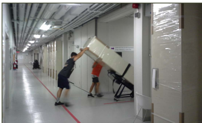
Figure 4. Movers using a tilting dolly to fit the new cabinets through low doorways.
