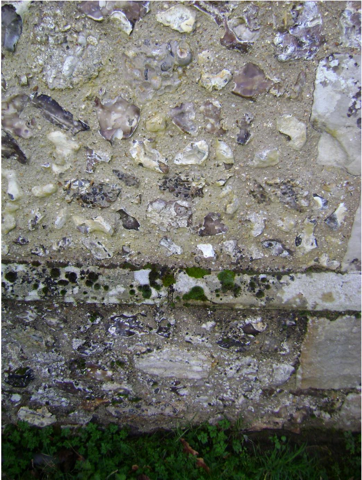
The chamfered limestone ledge running around the church walls is very mossy in places.
