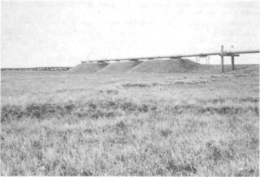
Fig. 2. Looking south along the 24-inch culverting constructed to simulate the transit-feeder pipelines proposed for use at Prudhoe Bay. Gravel embankments and wooden piling supports give an 8 and 5-foot clearance, respectively, in the underpasses, considered sufficient for passage of caribou beneath the obstruction.
