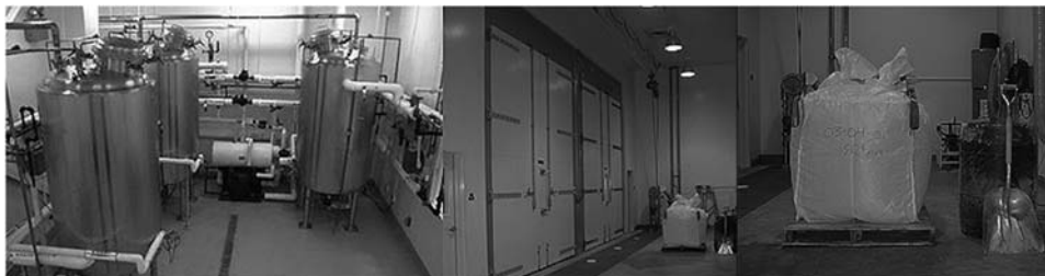
FIGURE 11.4 The 1990s Mycotech Corp. solid substrate mass production system for its Beauveria bassiana . (Left) Fermentation tanks for the production of inoculum for subsequent solid substrate phase; (Center) Two fermentation chambers (note large shovel for scale); (Right) Harvested B. bassiana conidia from one fermenter run, totaling 232 kg conidia powder with a titer of 1.2 \times 10^{11} conidia/g.
