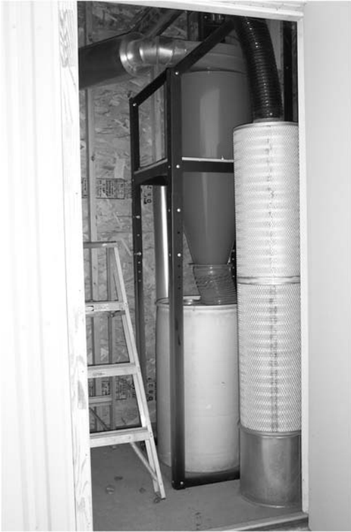
FIGURE 11.7 A cyclone dust collector, adapted from the carpentry industry, used to concentrate conidia mechanically dislodged from the solid substrate. The conidia are collected in the barrel beneath the conical collector. There is a HEPA filter on the exhaust to prevent the escape of conidia into the environment.
