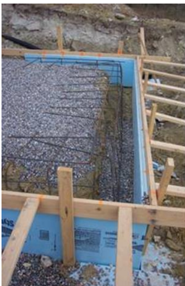
Above: Horizontal perimeter insulation partially installed and covered with earth.
