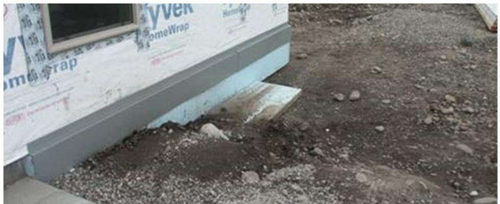
Above: Horizontal perimeter insulation partially installed and covered with earth.
