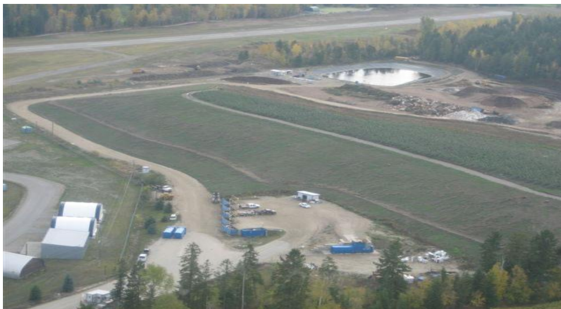
Aerial Photo of Award Winning project with phytoremediation poplar stand set up by Passive Remediation Systems Inc. on top of a land fill 132 .
