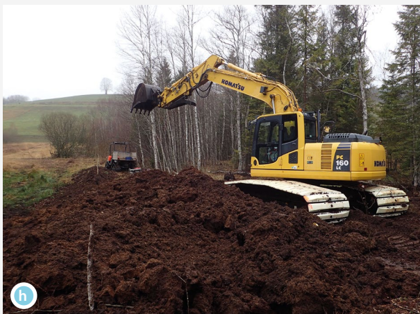
Consolidation works at the end of November 2018
