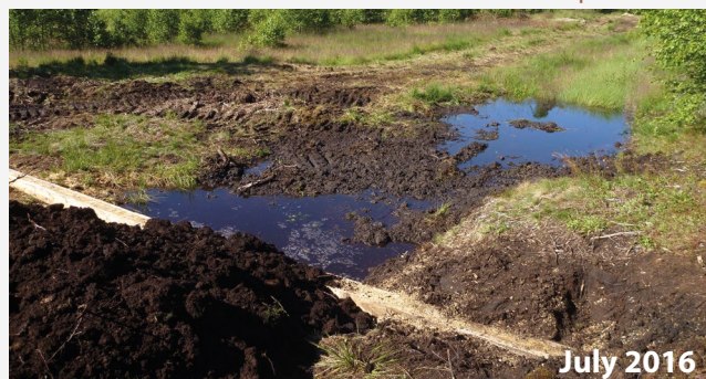
Complete obliteration of the ditch 6
