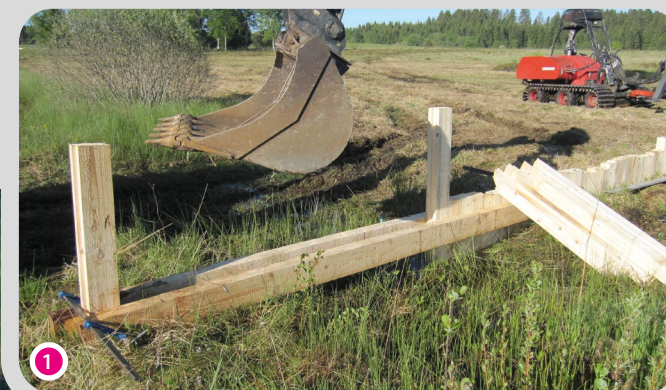
Installation of timber fences
