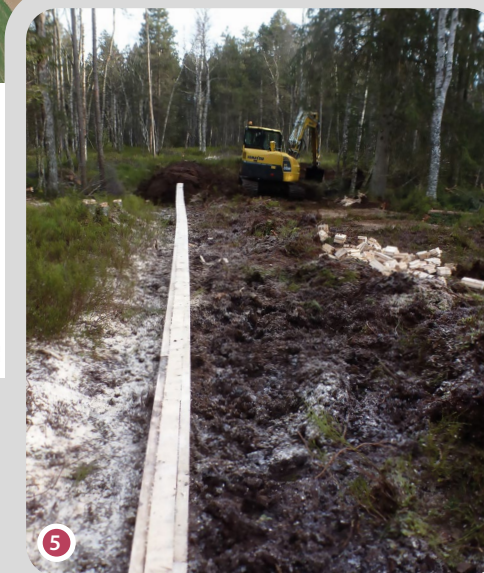
Covering of the timber plank fencing with peat and then vegetation
