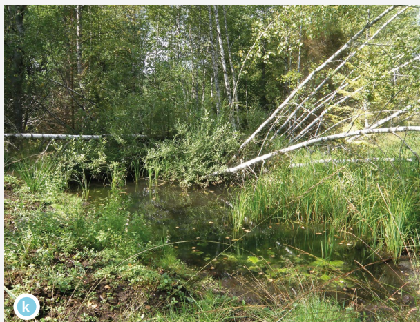
Downstream structure after two seasons of vegetation September 2019
