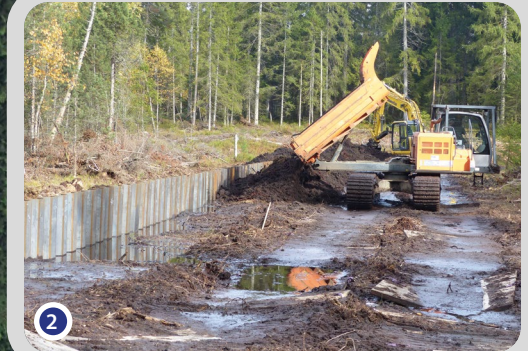
Metal topographical compensation dyke, covered with peat
