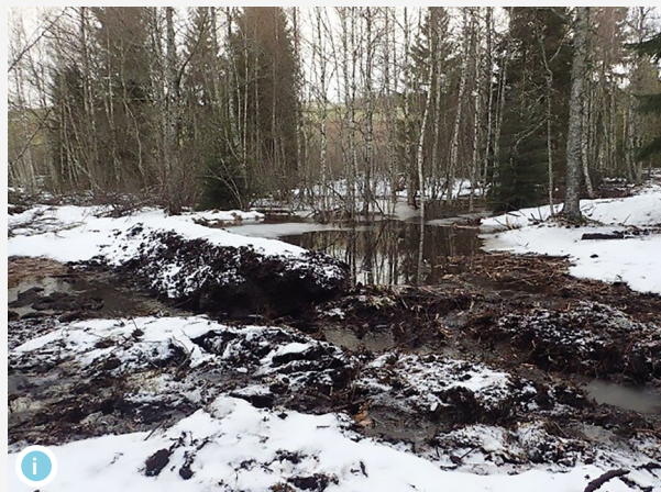
Erosion at the downstream dyke
