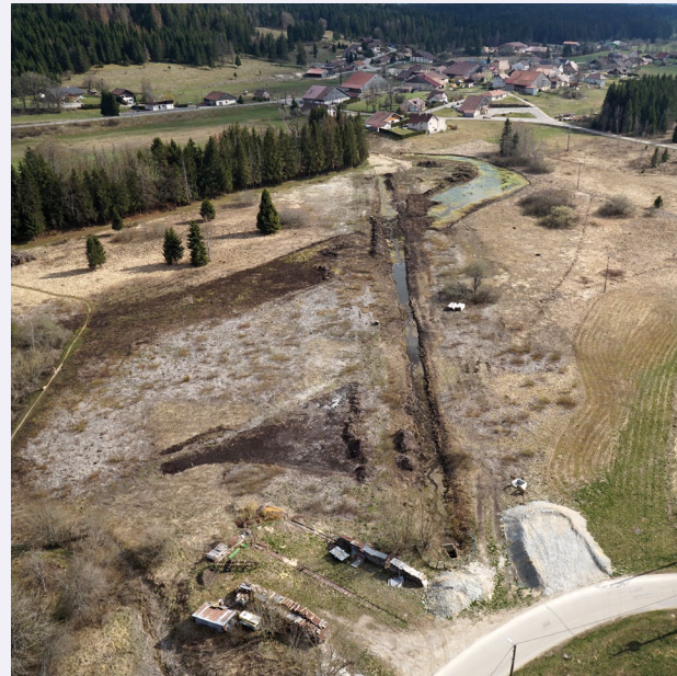
neutralisation of the drainage ditch in the Lac de Malpas peatland
