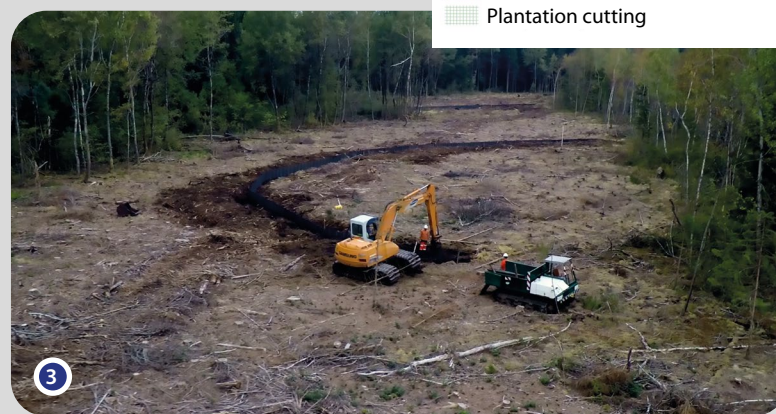
Dam no. 3 during construction
