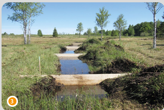
Step 1 in the ditch neutralisation: placing the wooden panels
