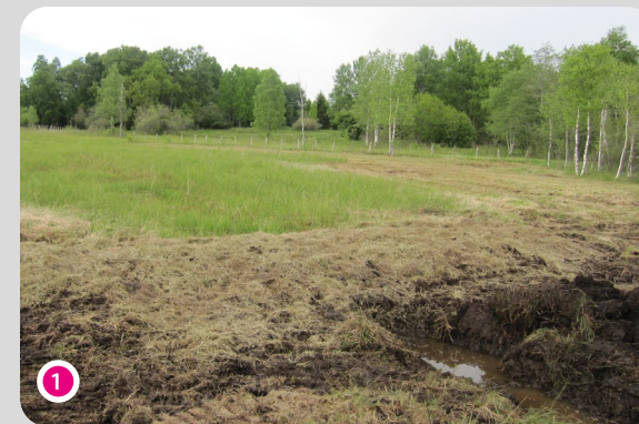
Upstream fence, covered with peat and straw
