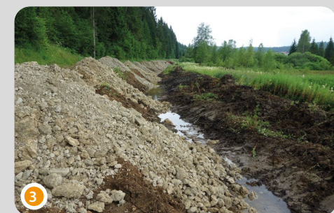
Moraine was chosen to fill in the south feeder drain as the volume involved was large, access was easy and the ditch was situated along the slope, therefore largely influenced by mineralised waters
