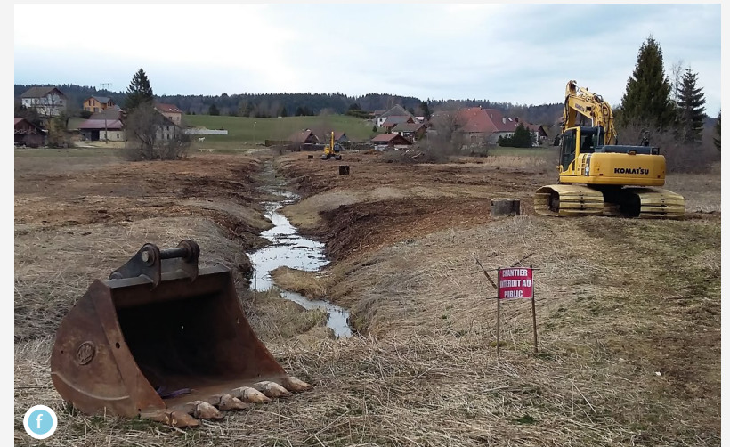
Central ditch in the peatland to the south of the Lac de Malpas after shredding of the willow stand and before neutralisation
