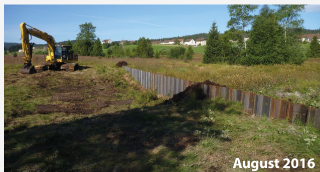
Rewetting of the old peat cutting pits by installing a fence 8
