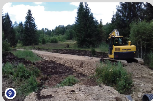
Moraine was chosen to fill in the south feeder drain as the volume involved was large, access was easy and the ditch was situated along the slope, therefore largely influenced by mineralised waters
