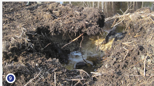
The overspill on the dyke very quickly generates a breach by erosion
