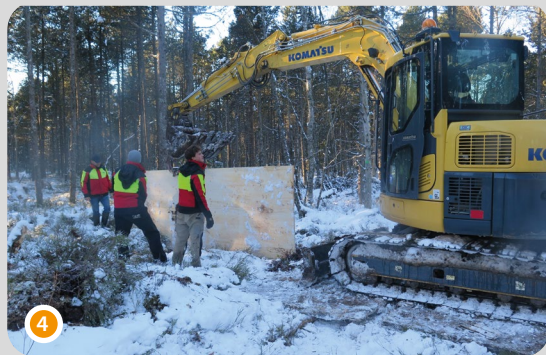
Installation of three-ply fence panels
