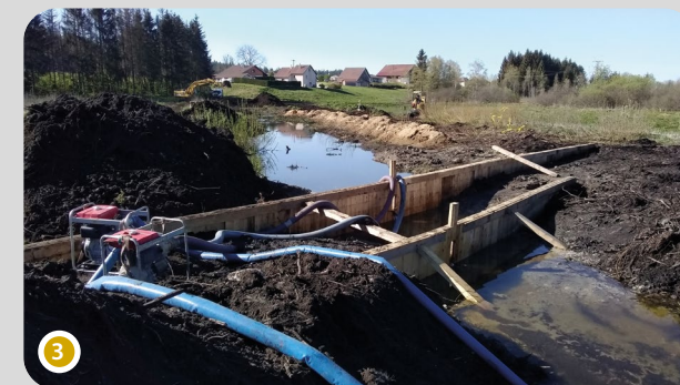
Construction of the double fence on the central ditch
