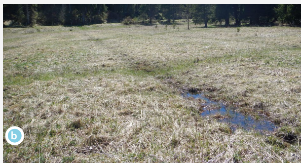
Ditch before the works
