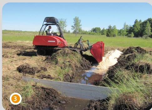
Step 2 in the ditch neutralisation: filling the channel with sawdust
