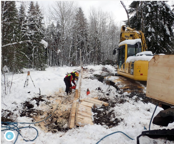
Work being carried out in unfavourable weather conditions
